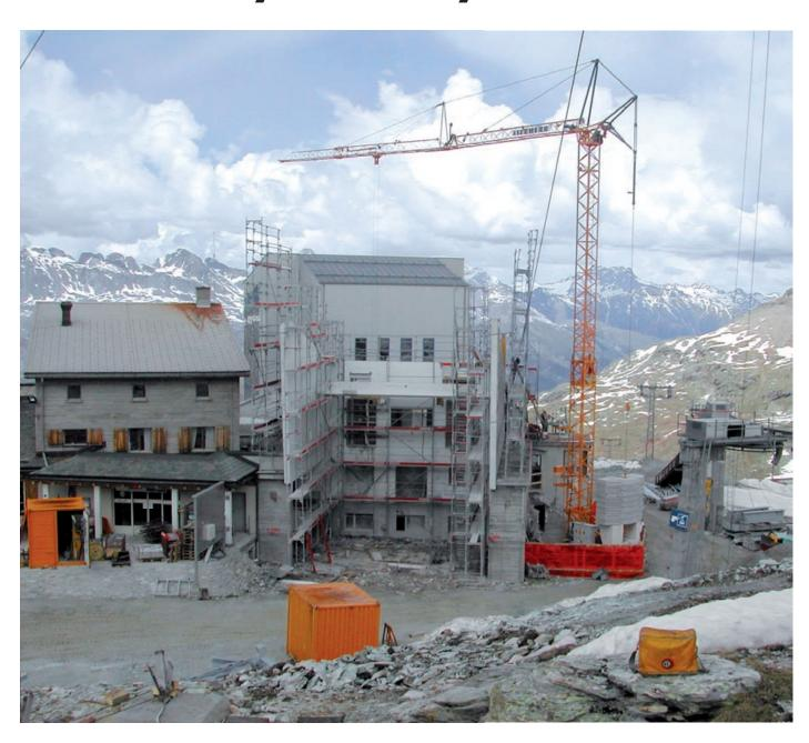
The Murtèl mid-way station on Piz Corvatsch is being extended by the construction company Nicol. Hartmann & Cie. AG at an altitude of more than 2,700 metres, and a Liebherr 34 K fast-erecting crane is hard at work.
