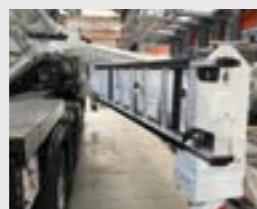
Ladder to fuel tank access
